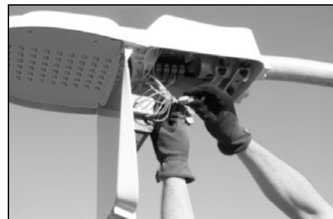
Removable "power door" opens without tools and hangs securely during wiring.
