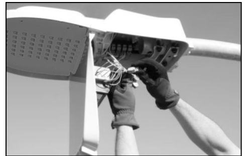
Removable "power door" opens without tools and hangs securely during wiring.
